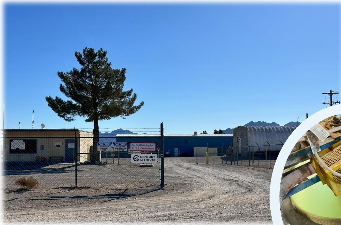
Demonstration Plant Facilities
